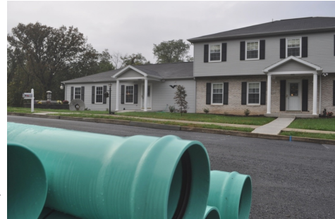
The pipes before the trenching
